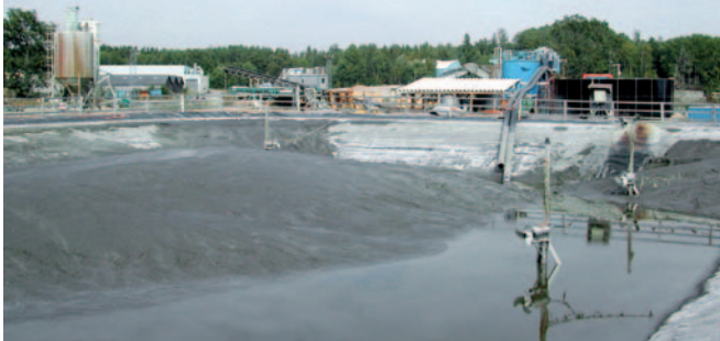
The dredger (above, left) in action in the bay. Below it is a sedimentation tank for the dredging spoil. The picture above shows the dewatered screenings being laid up inside the newly constructed retaining wall.
